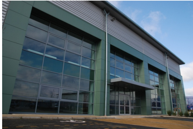
Virtus's 8MVA Enfield site
